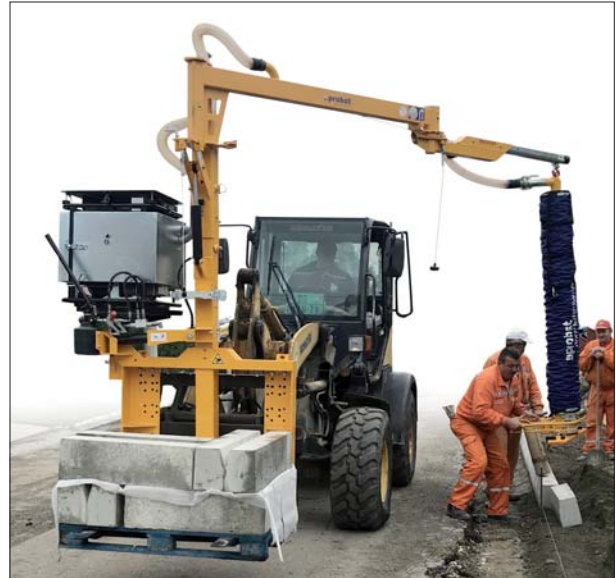
JUMBO-BV-VARIO Vacuum Kerb Stone Installation
