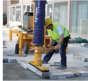
JUMBOMOBIL JM-VARIO Vacuum Slab Laying Machine
