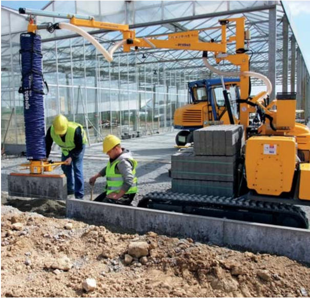
TRANSMOBIL TM Installation Carrier installing kerbs
