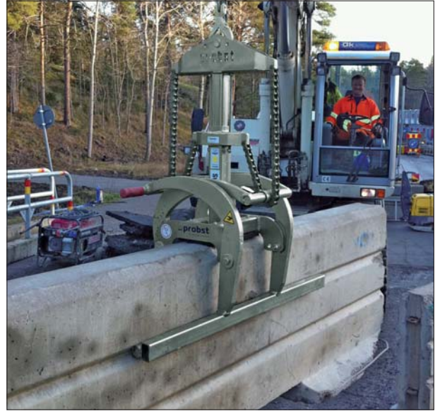
Grab for Prefabricated Concrete Products FTZ-GBA-S
