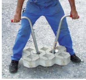
Turf Stone Handles RVH
