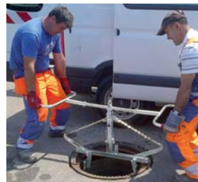
Manhole Frame Clamp SRZ-M
