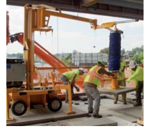
JUMBOMOBIL JM-VARIO Vacuum Slab Laying Machine
