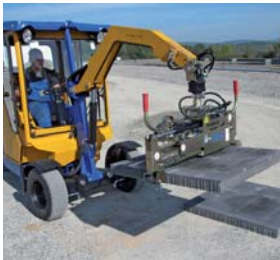
Hydraulic Laying Clamp VZ-H-UNI
