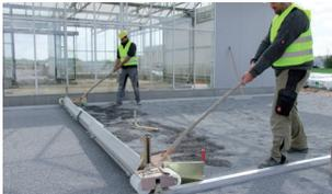
Precise laying course adjustment due to height-adjustable, smooth-running roller units with guide plate and folding deflector.
