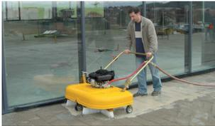
Fast & inexpensive filling of pavement joints on small and medium sized areas. Joint material can be grouted dry or wet.
