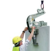
Exact placement of L-stones: Suspension eye can be adjusted to the centre of gravity of common elements so that they hang vertically.
