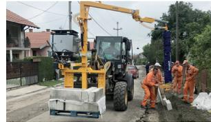
Vacuum kerb lifter with innovative safety features: lay kerbs quickly, safely and ergonomically.
