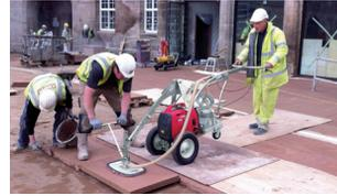
Complete unit for rapid vacuum laying of highly porous laying materials such as natural and concrete stone slabs.
