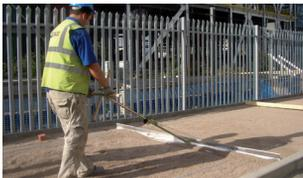
Hand tool set for the efficient screeding of small and medium sized subgrade surfaces: time-saving and ergonomic, all without kneeling.
